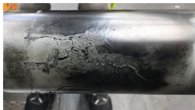
Fig. 7: Fault location inside the joint. It is clearly seen that the fault was located correctly even though it was not possible to visually confirm on the outside of the joint.
